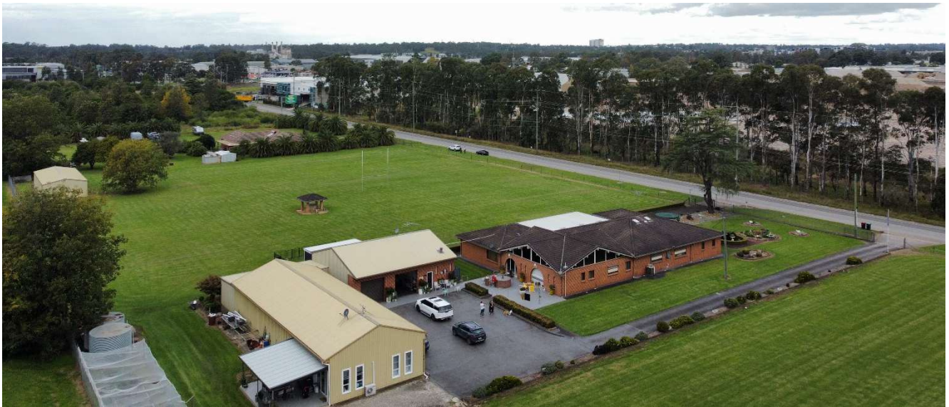
Figure 2. Modified floodplain landform within the project area (Morson Group 2024)
